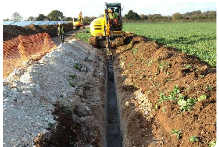
Cable trenching, showing topsoil stripped and set to one side, with subsoil placed on the other side ready for reinstatement (photo courtesy of British Solar Renewables)
